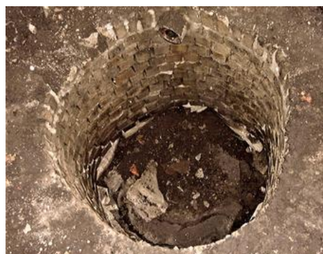
A dried up well, caused by lowering groundwater levels.
